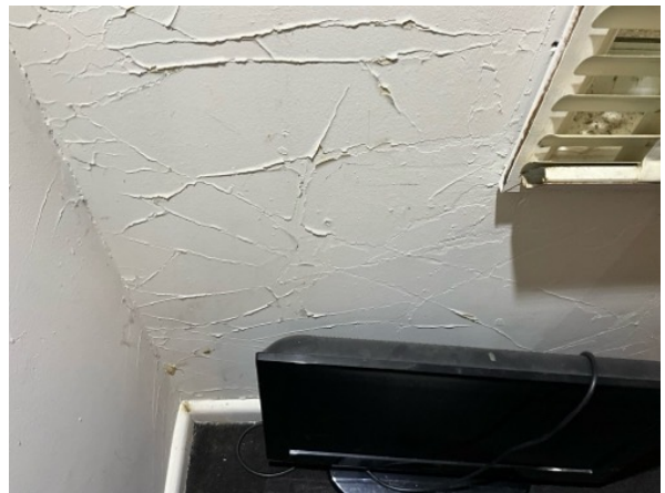
Plaster finishes have numerous cracks and deficiencies observed
