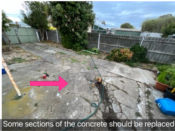
Significant cracking and movement observed to the concrete
