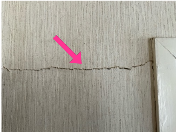
Numerous cracks observed to the plaster finishes throughout the home
