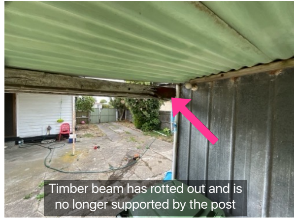
This roof has not been built to recognise standards with beam spanning excessive distances
